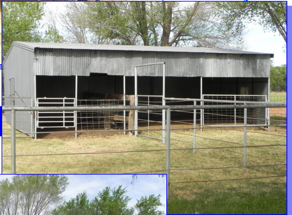
RV Port, Barn & Pens
